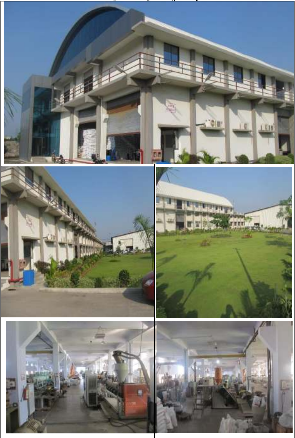
Photos of our Manufacturing Facility-1
